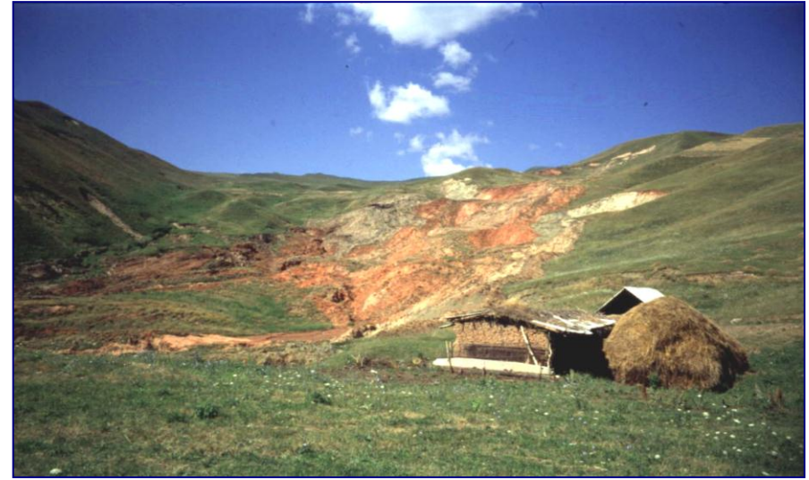
Displacement of clay-rich tertiary sediments during period of several days in June 1998
